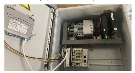
The **WAN port** is reserved for the customer's network so the CAL-EDGE-0 device can access the Internet. So it is essential to connect that Ethernet cable in the WAN port.
