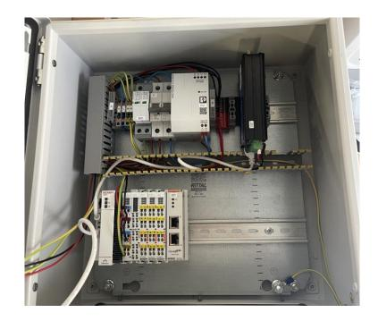
The router is supplied with 24VDC, so to power it, the red wire needs to be connected to a 24VDC terminal from the terminal block and the black wire needs to be connected to 0VDC terminal from the terminal block like shown in the photo.
